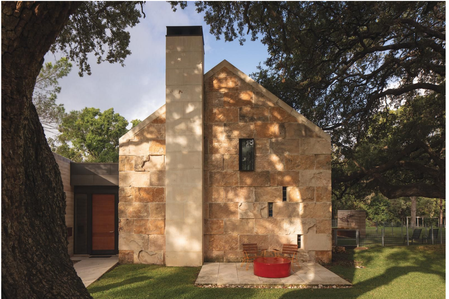
The shape of the main stone facade is the classic gable shape that a child might sketch when asked to draw a house, explained Harrison. "I am drawn to iconic shapes that present a clear illustration of the spaces contained within," he said.
